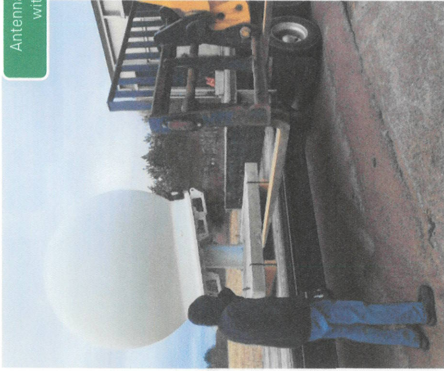
Control tag lines are recommended for overhead lifts
